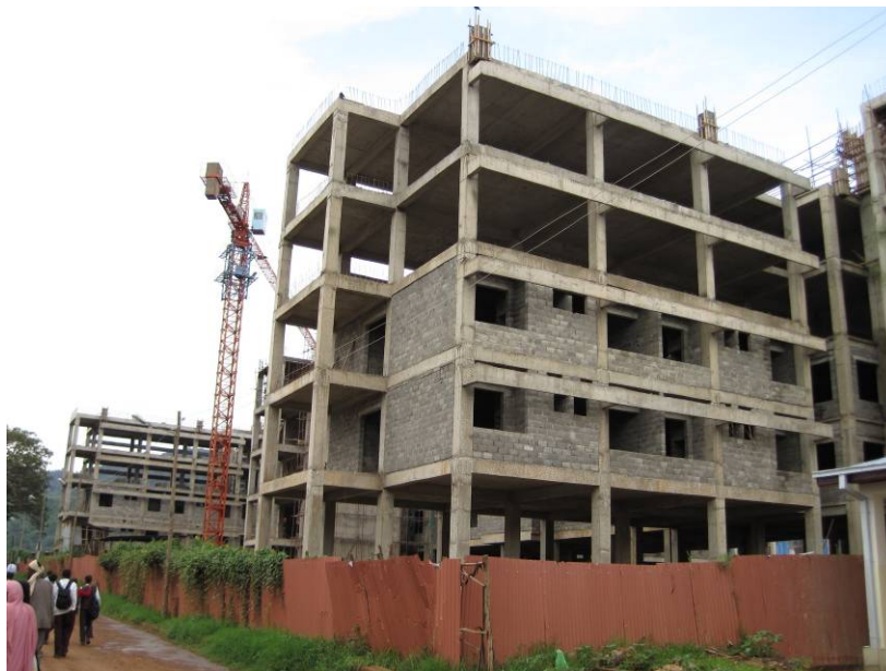
Fig. 8 JU New Hospital Construction
